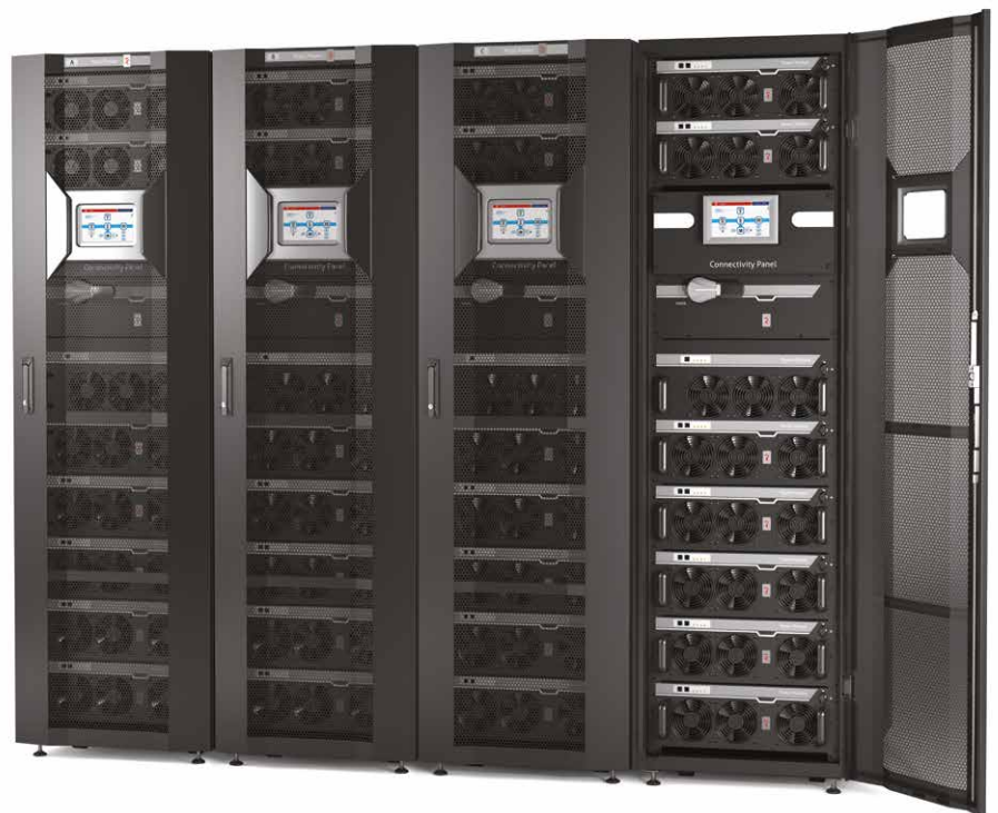
Power Cabinet (1÷7 x Power Modules) x 4
